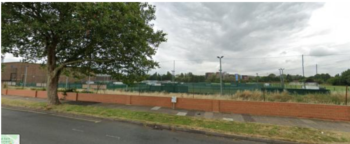
Fig 10: Existing views of Site from Copers Cope Road (existing Gambado building on left) (Credit: Google Maps)
